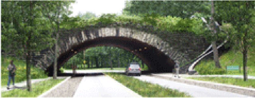
PROPOSED WEST PARK AVENUE BRIDGE RESTORATION
